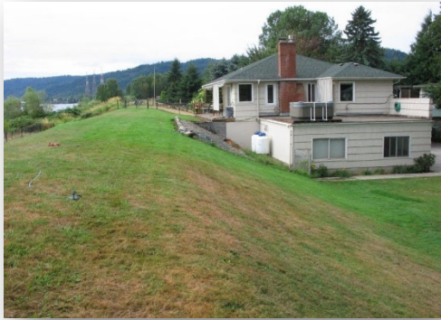
FIGURE 7-10: UNACCEPTABLE LEVEE ENCROACHMENT BY HOMEOWNER
